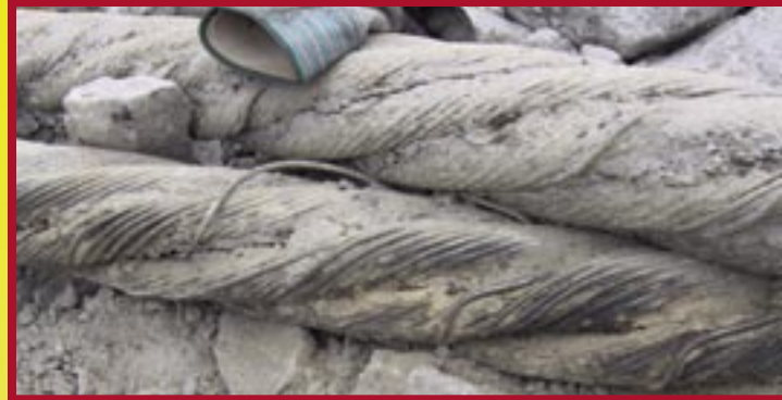
Figure 2: Severely Deteriorated Wedge
